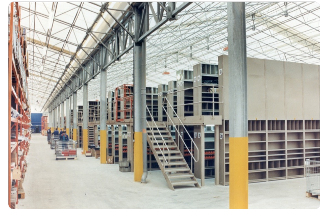
Mezzanines and/or modular office spaces
